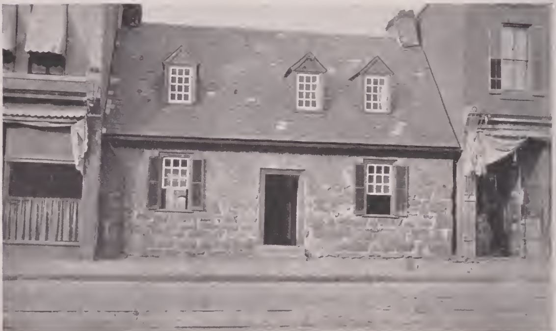
Old Stone House, Richmond, the oldest in the city, now a memorial to Edgar Allen Poe.
